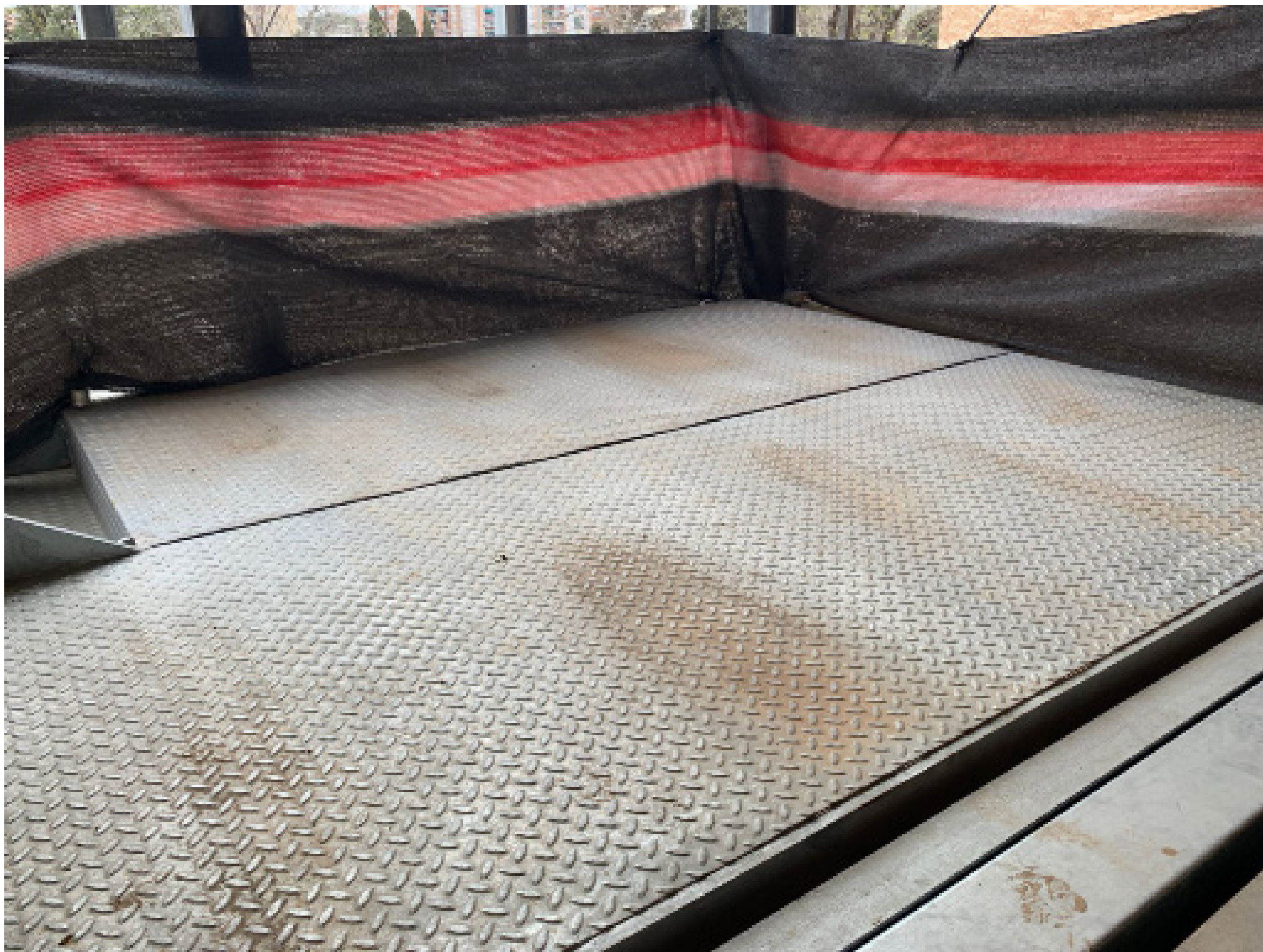
Refer xapa replans ESCALA 1,2 i 3 per abombament.
