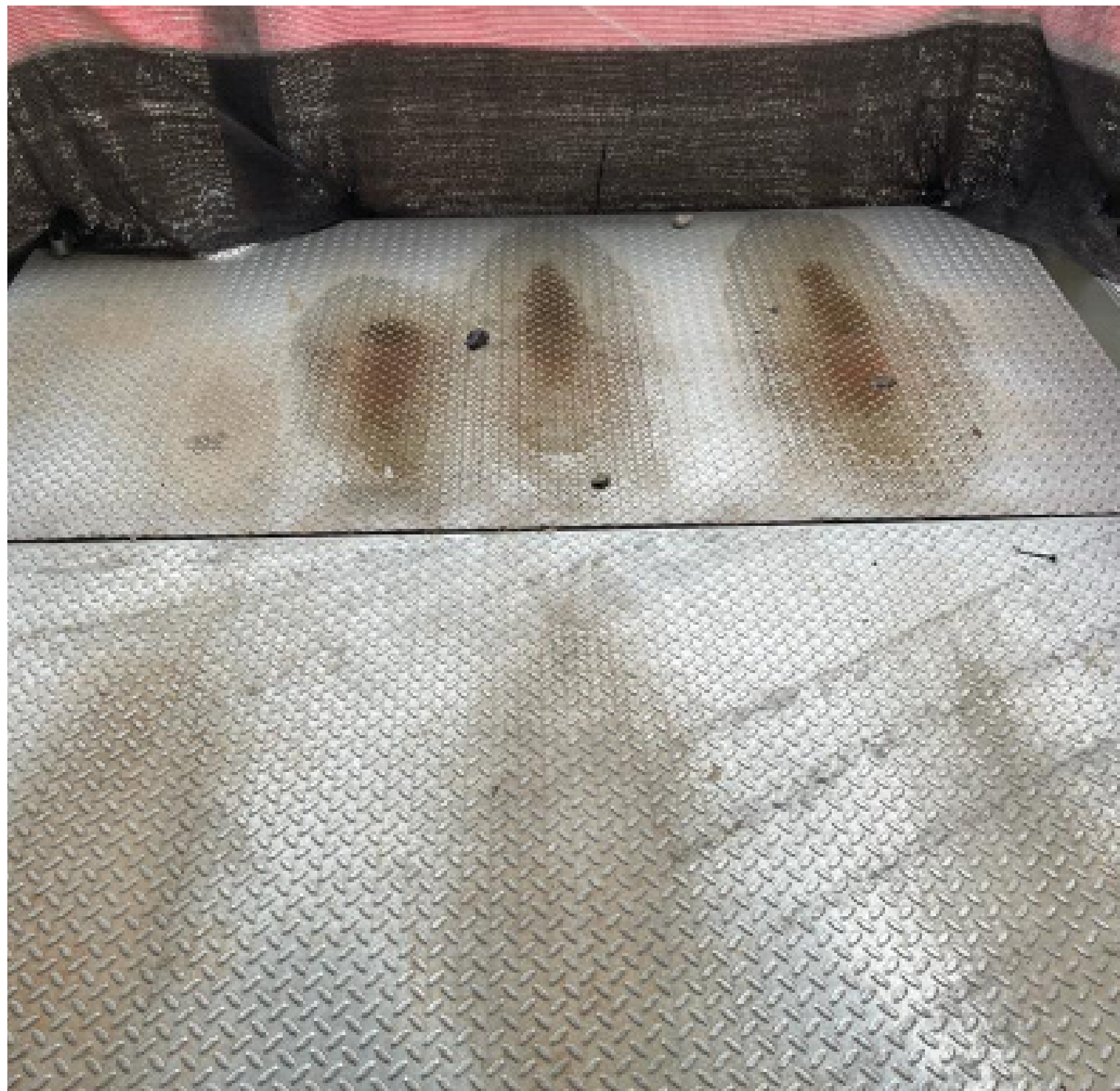
Refer xapa replans ESCALA 1,2 i 3 per abombament.
